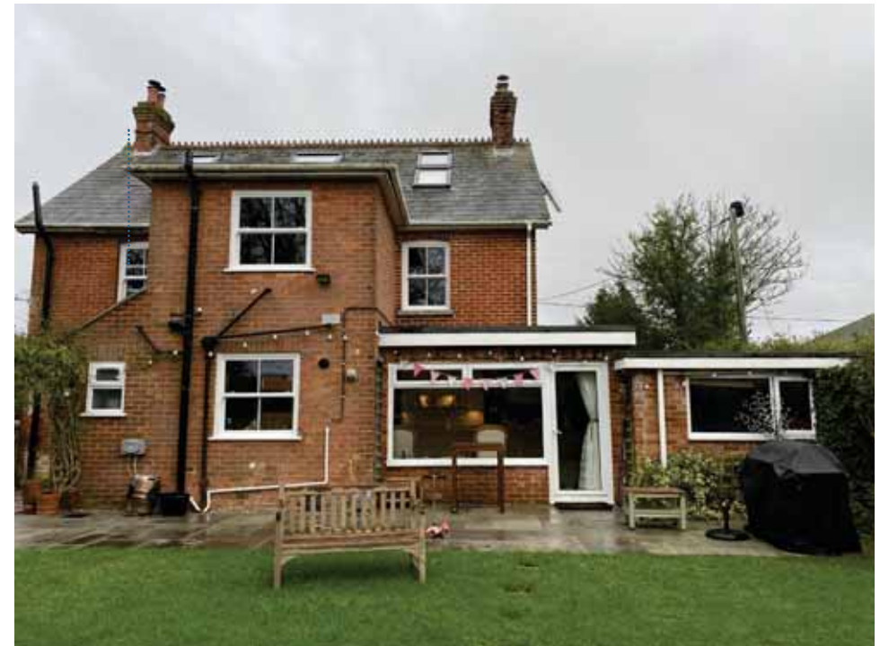
Photograph of the existing rear elevation
