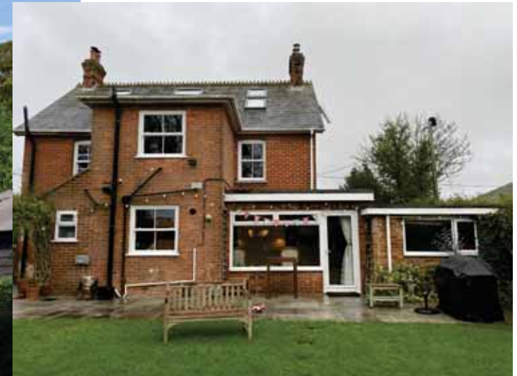
Photograph of existing rear extensions.
